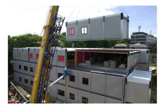
Volumetric offsite construction reduces the production of waste to 1.8% through efficient design, continuous process improvement, involvement of the supply chain as well as procurement strategies and, ultimately, erection on site.
