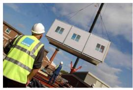
In North America and Europe, volumetric (modular) construction has been associated with temporary buildings. These temporary buildings had to be rapidly built and delivered, with a minimum disturbance on site. Manufactured modular buildings were perfectly suited for these purposes and were adopted as temporary structures.
