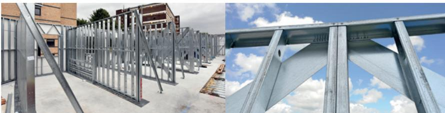
***"We had very early involvement in the design of the building, but manufacturing and installation took just 16-weeks. The on-site erection of the offsite manufactured light steel wall panels (with factory installed weather defence board) and floor cassettes (with factory installed steel decking) was completed 14-weeks ahead of the original 30-week target installation program."***
