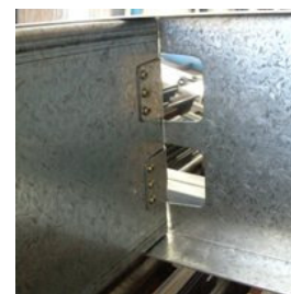
Joist Connection
